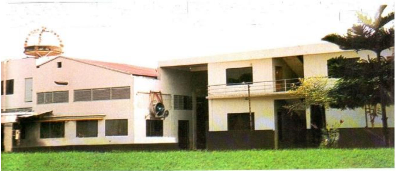
Picture-2: Front View of the Fabric Dyeing Dept.
